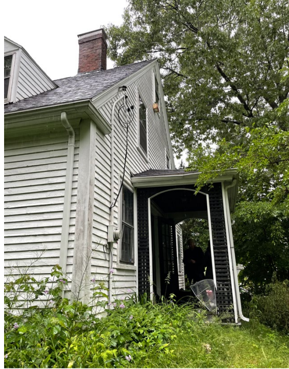
Figure 5: East facade and entry porch. Photograph taken June 9, 2022.
