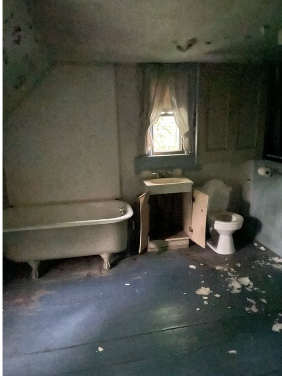
Figure 15: Second floor southwest bedroom (converted to bathroom). Photograph taken June 9, 2022.
