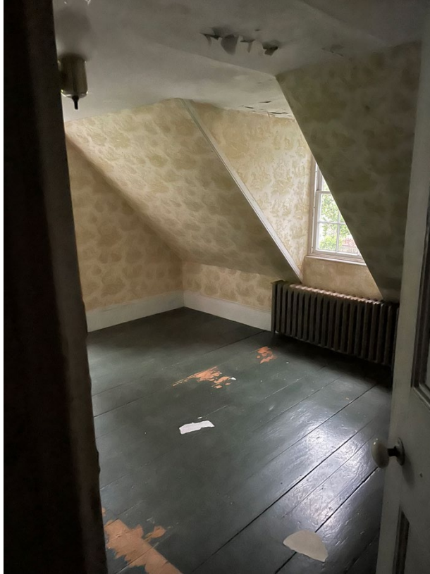
Figure 17: Second floor, southeast bedroom. Photograph taken June 9, 2022.
