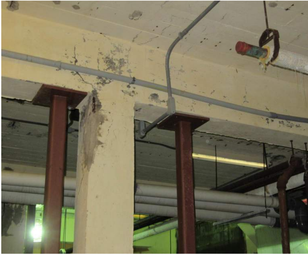
Photo 5: Typical Shoring - Filtration Room Roof Beams
