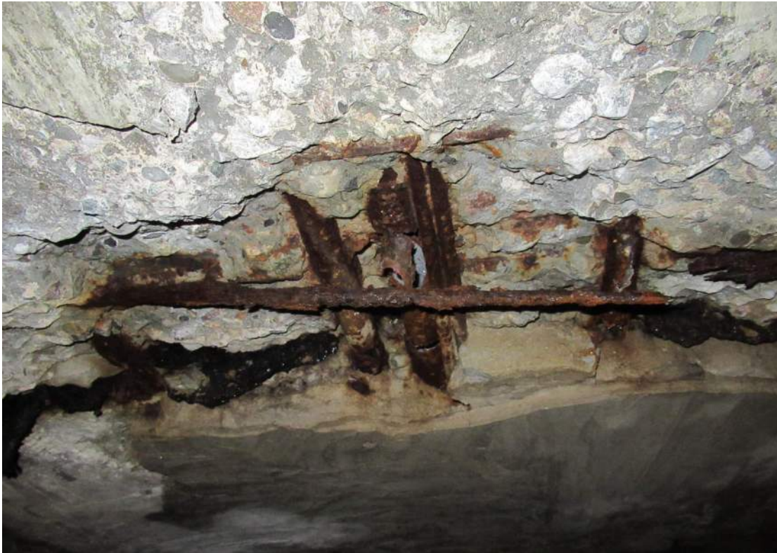
Photo 9: East Tunnel Concrete Ceiling Spall Requiring Shoring
