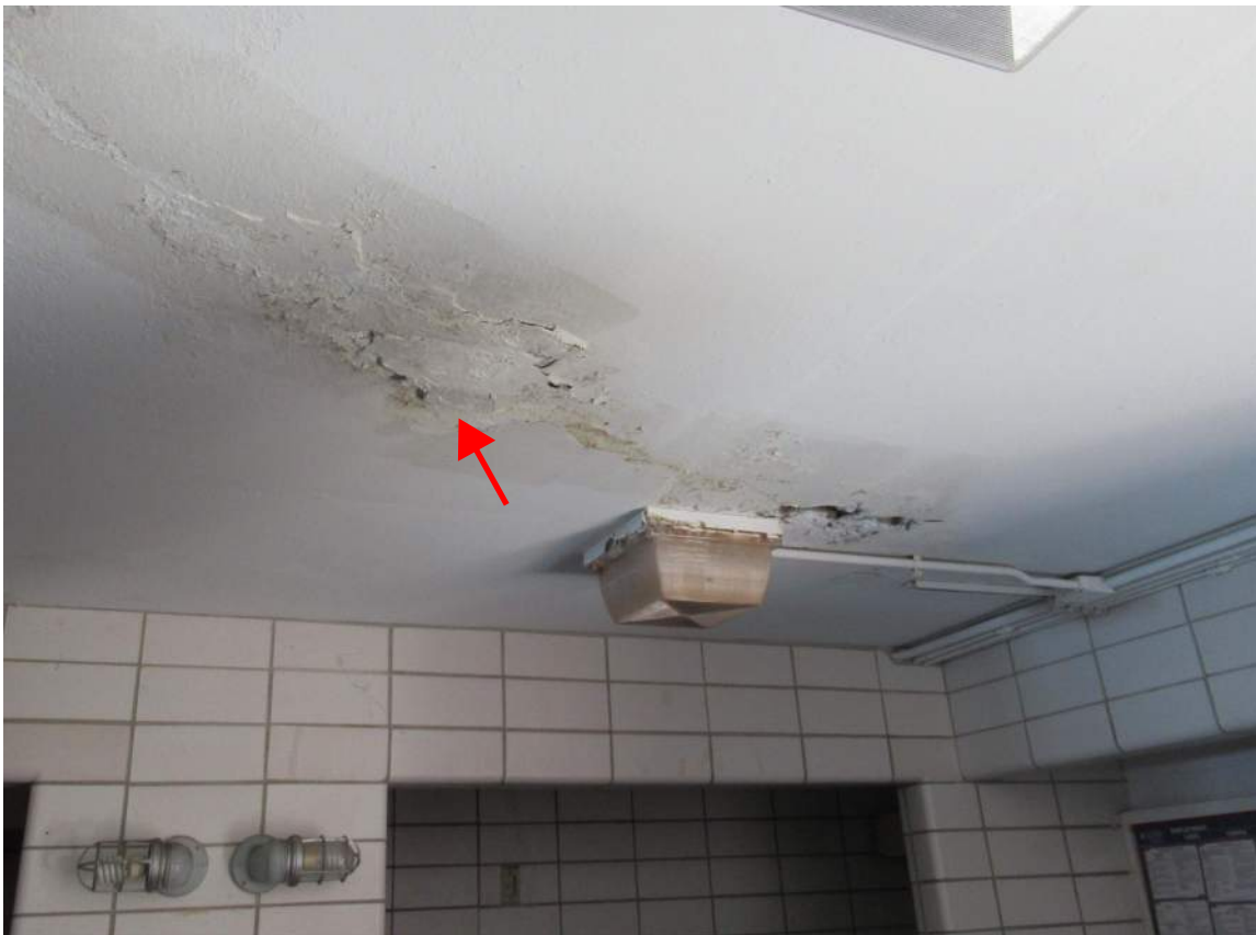
Photo 9: East Tunnel Concrete Ceiling Spall Requiring Shoring
