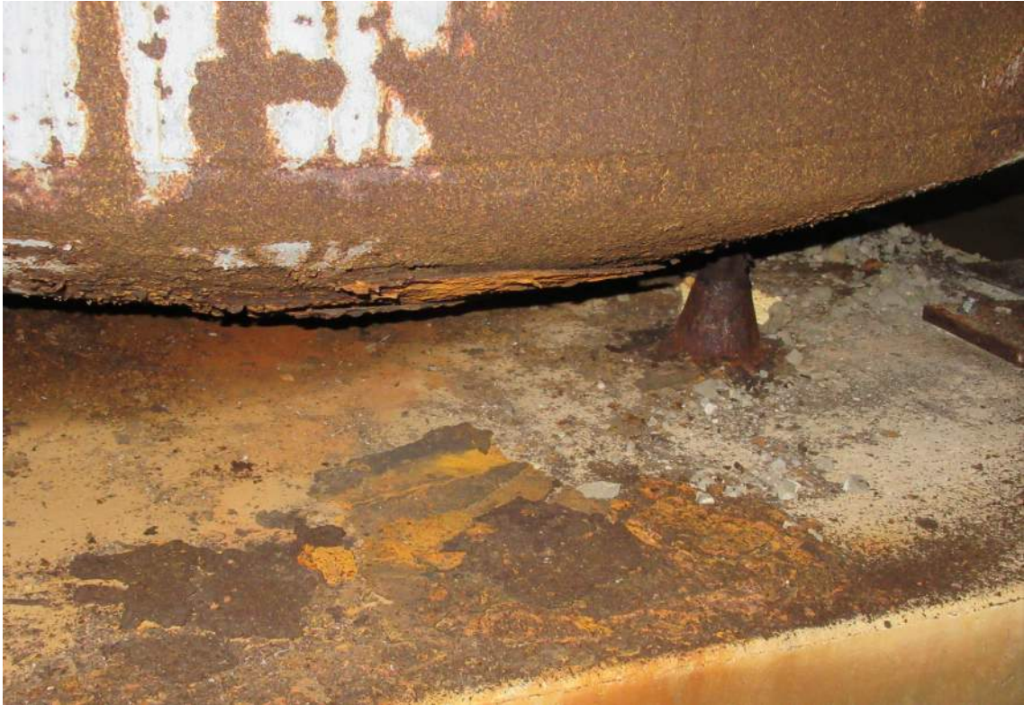
Photo 7: Concrete Spalls Ceiling of Men's Changing Room, Bathhouse
