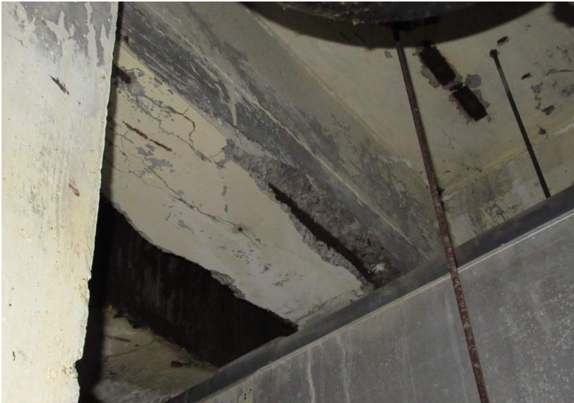
Photo 8: Filter Room Concrete (Double) Beam Requiring Additional Shoring
