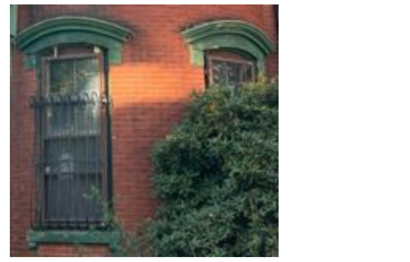
PHOTO 1.1 - REPLACE WINDOW (REFER DETAIL 5) RETAIN/ REPAIR LINTEL AND SILL, PAINT FINISHED (SEE NOTES)
