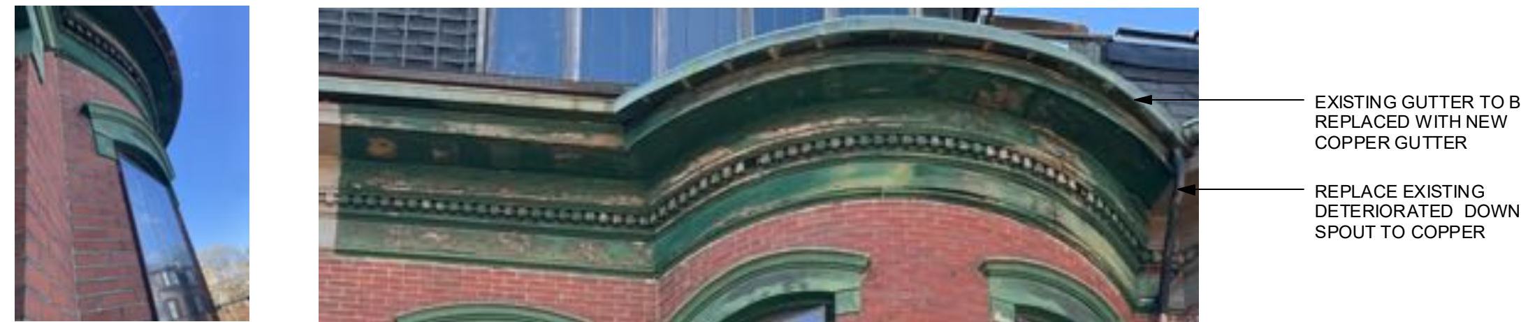
PHOTO 3.2 - RETAIN, REPAIR BROKEN PIECES AND REPAINT EXTERIOR TRIM
