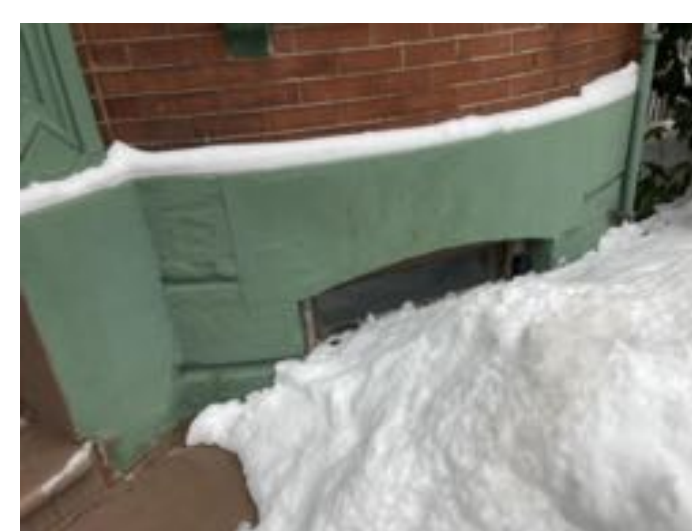
PHOTO 1.1 - REPLACE WINDOW (REFER DETAIL 5) RETAIN/ REPAIR LINTEL AND SILL, PAINT FINISHED (SEE NOTES)
