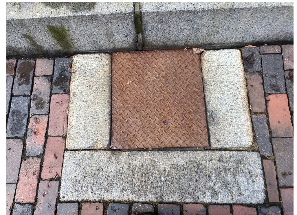
LOUISBURG SQUARE TYP. COAL CHUTE PRECIDENT
