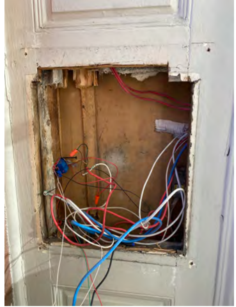
Existing Cutout in Paneled Entrance Surround; Former Intercom Cut into Width of Stiles and Rails; Outline of Larger Base Plate Visible at Perimeter
