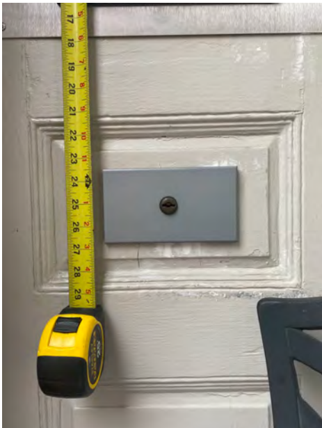
Detail of Intact Raised Panel and Moulding Below Intercom; Gray Box for Letter Carrier Access
