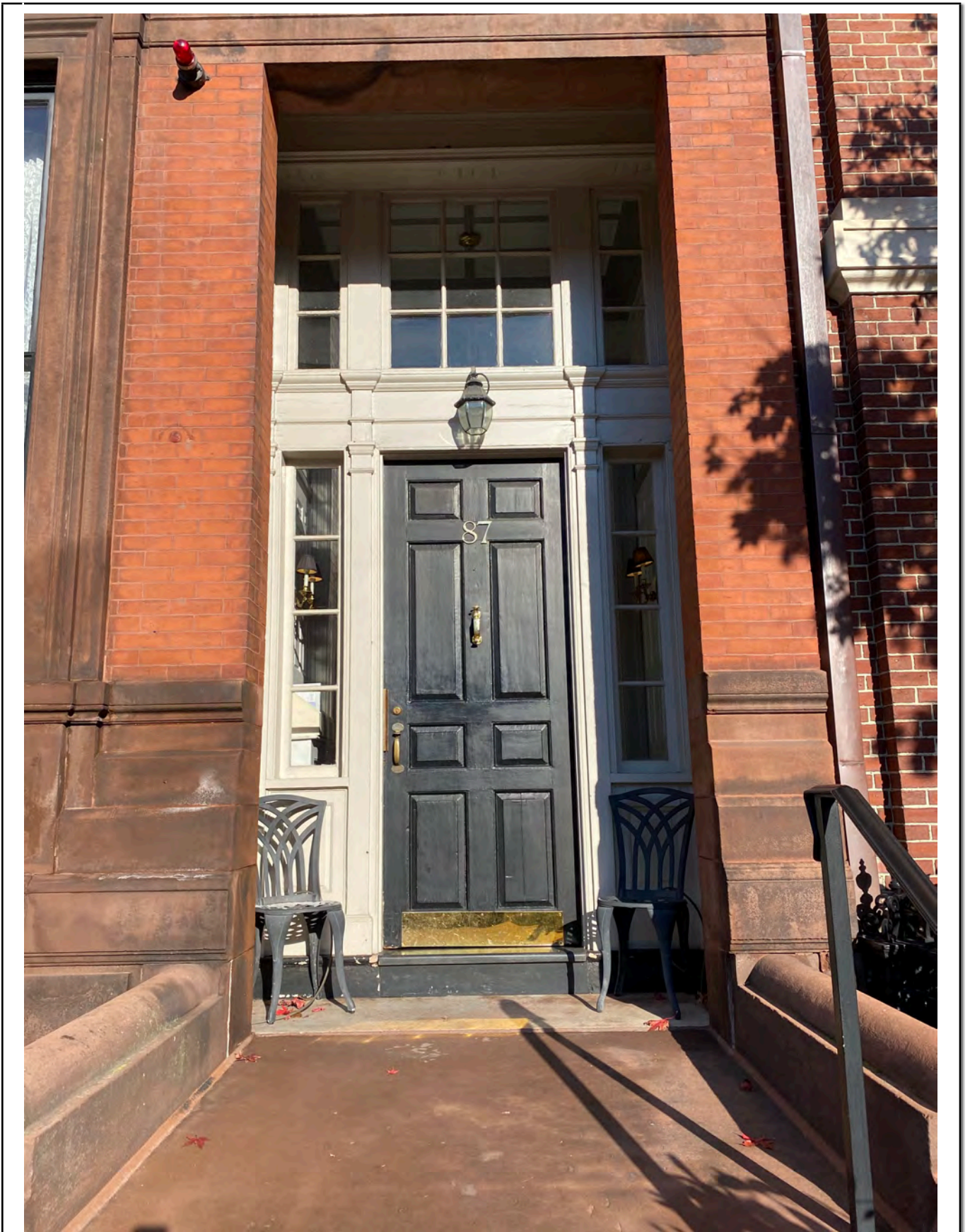
Walkway to Front Door and Entrance Surround at 87 Beacon Street Across from Public Garden
