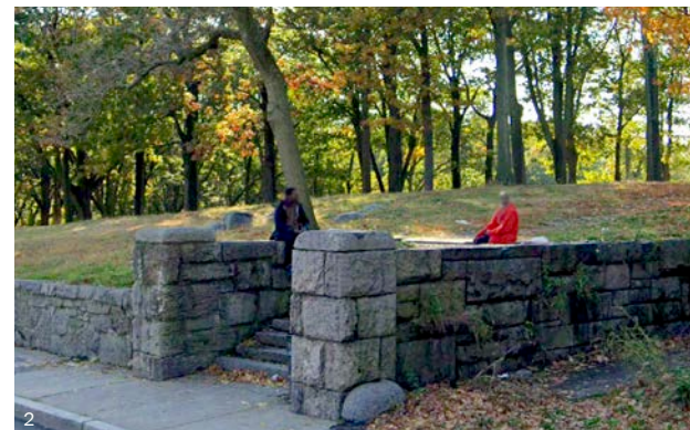
Medium Entrance: Historic stone masonry at the old Refectory.
