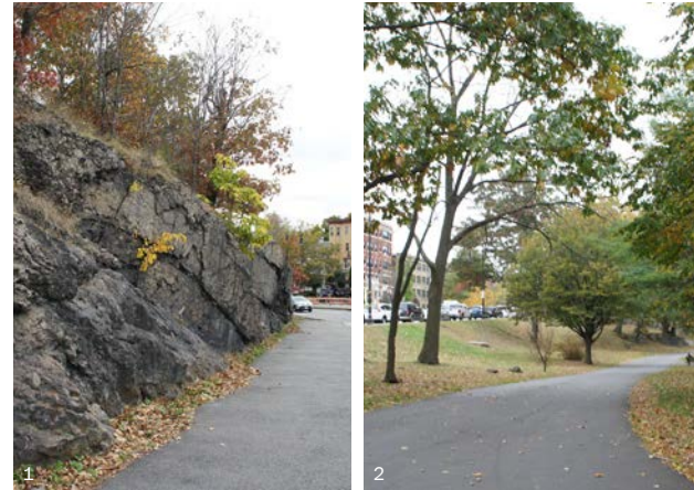
The varied edge conditions along Seaver Street.
