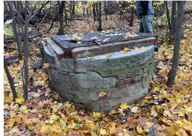
The existing outlet control structure at Scarboro Pond
