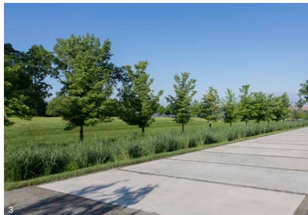
3 Vegetated swale at the edge of parking.
