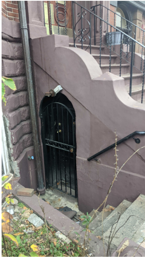
EXISTING STOOP SIDE ENTRY
