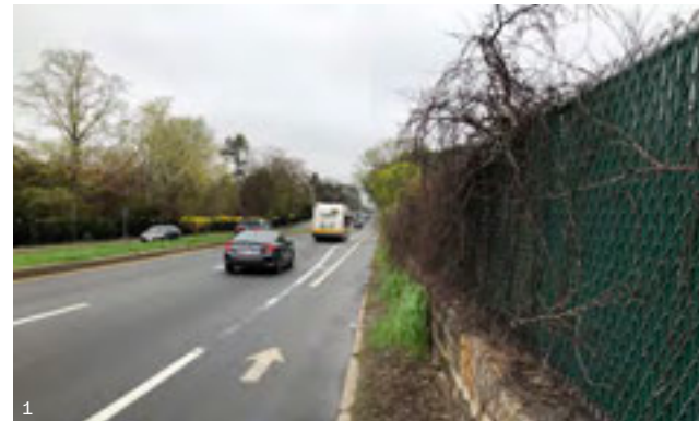
1 The low historic puddingstone perimeter wall with a chain link fence and no sidewalk along Morton Street, a state highway.
