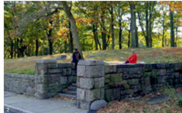
2 The existing entrance on Blue Hill Ave between McLean and Charlotte Streets.
