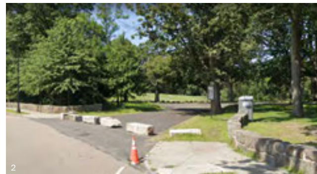
2 The historic carriageway entrance with granite boulders used to block car access.
