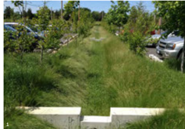
1 Vegetated swale in the center of parking.
