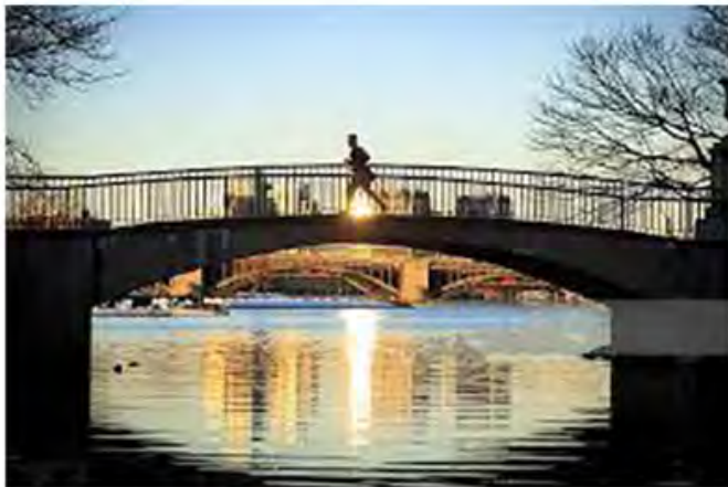
Bridge on Boston Esplanade - Arthur Shurcliff
