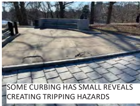
CONCRETE PAVING SETTLED, CREATING TRIP HAZARD AT BACK OF CURB
