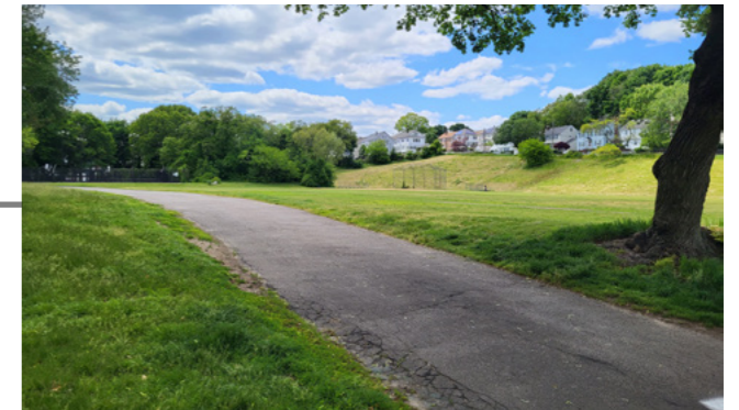
Asphalt Main Path
