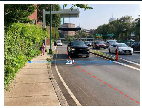
Above: a red dashed line shows where the approximate edge of a 10 foot wide path would be. A blue solid line shows the narrowest constrained dimension in the Storrow onramp area.
