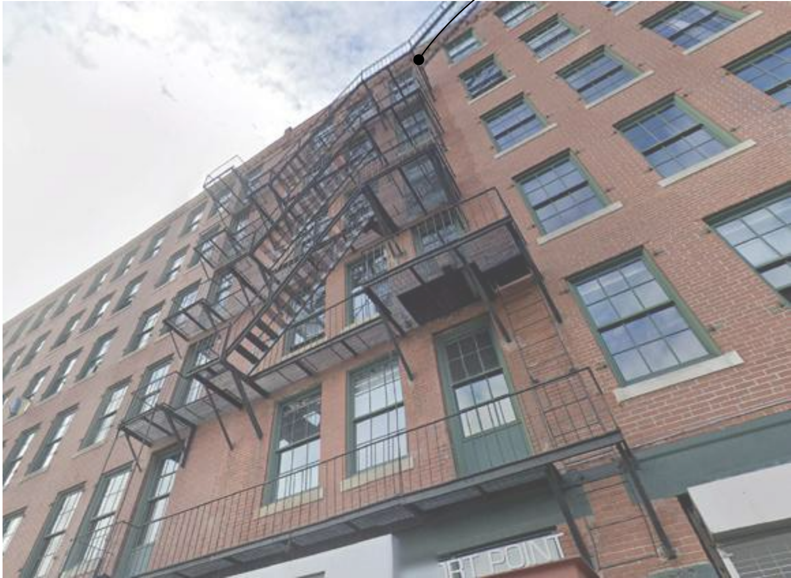
15 Channel Center - Medallion Ave. Facade
