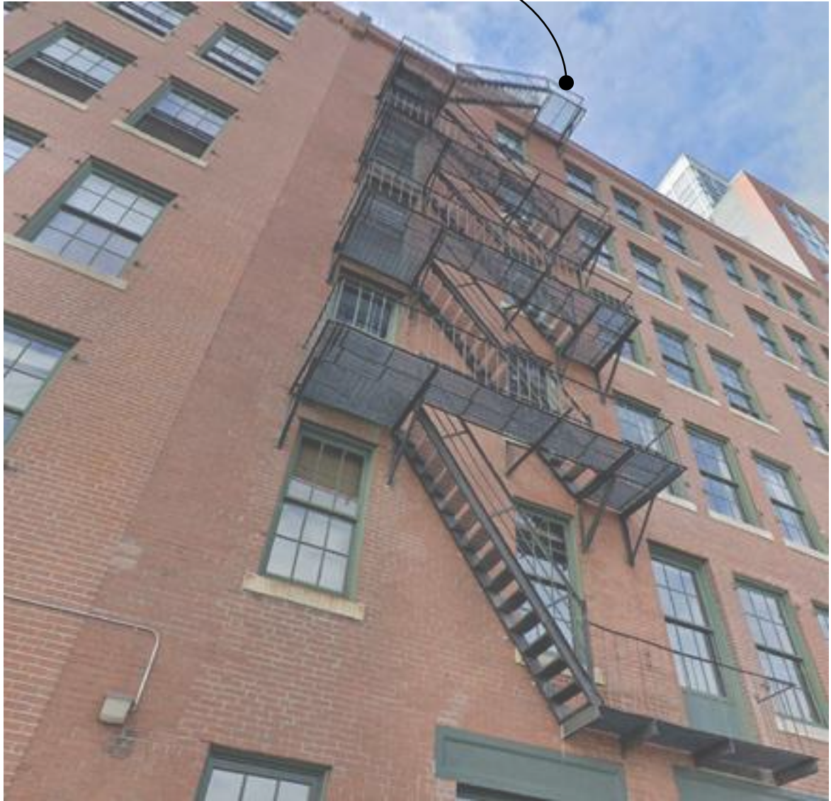
15 Channel Center - Medallion Ave. Facade
