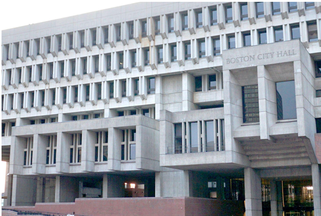
Figure 11. Cast-in-place concrete hoods for City Council offices (left) and City Council Chamber (right). (2023)
