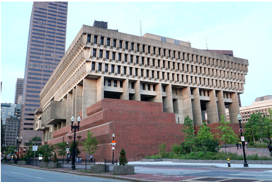
Figure 6. Brick terracing at the northeast corner of the building. (2023)
