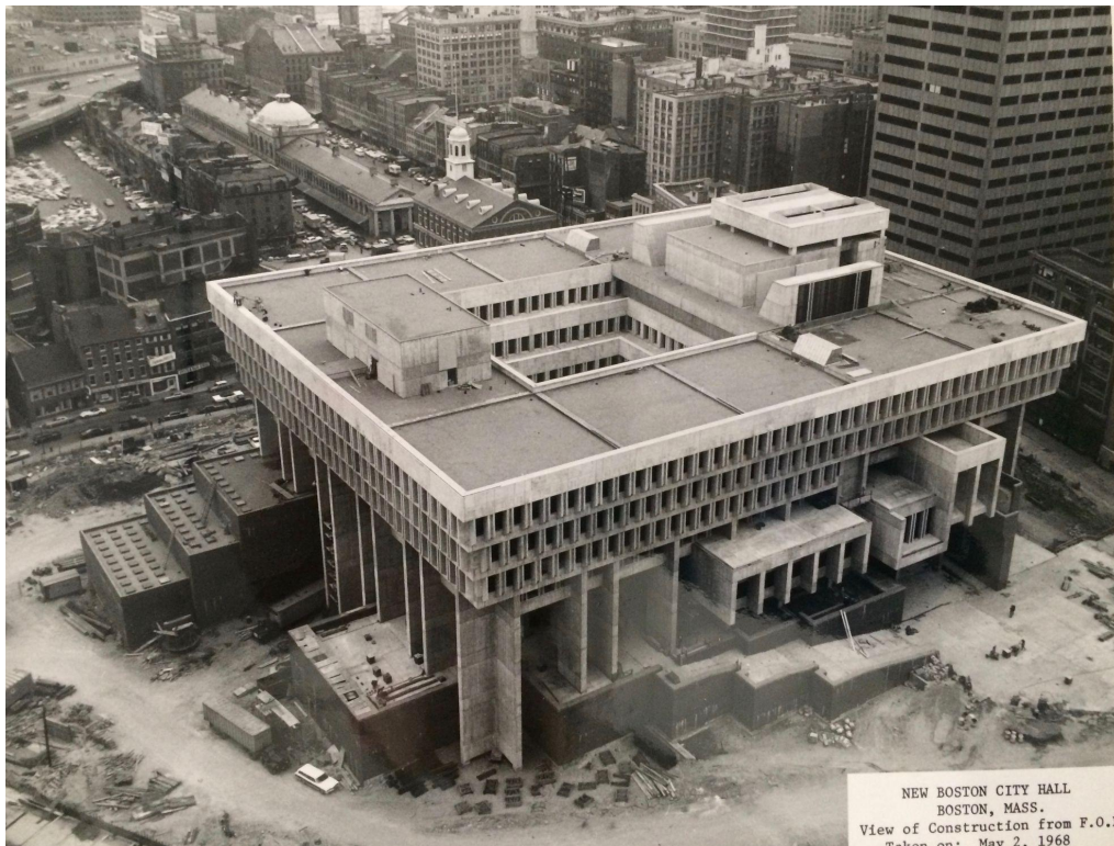
Figure 18. Boston City Hall under construction; looking southeast from JFK Building. (1968)
