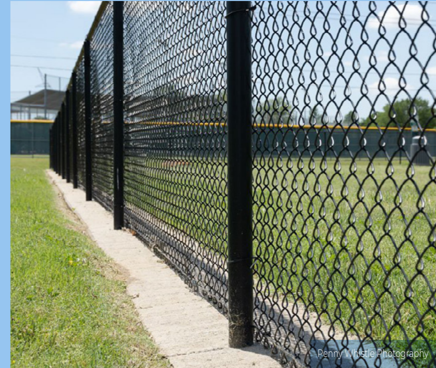
New Fence with Concrete Mow Strip at Clancy Road
