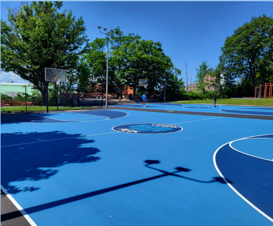
Renovated Basketball Court
