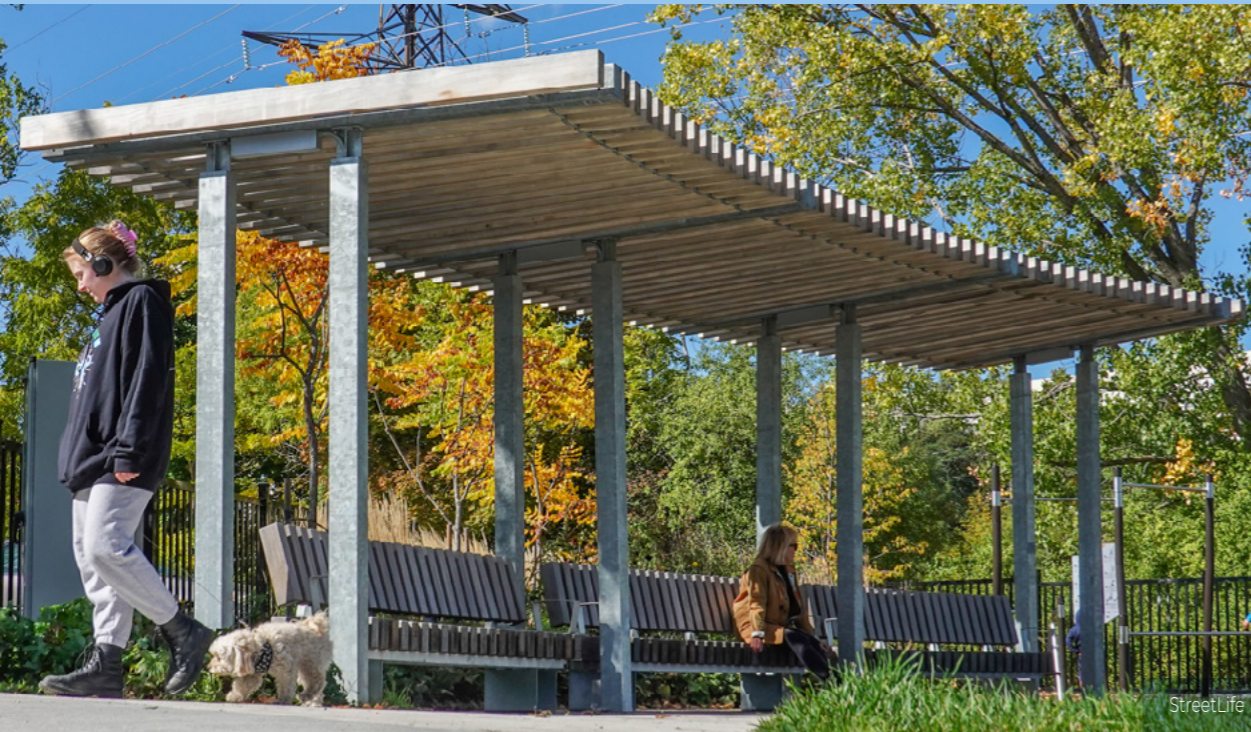
Curved Shade Structure
