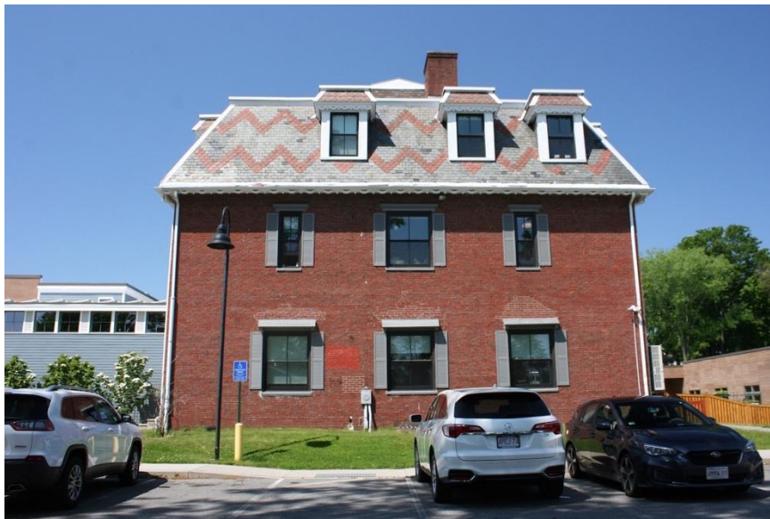
Figure 11. East elevation. Photograph by Wendy Frontiero, June 2023.
