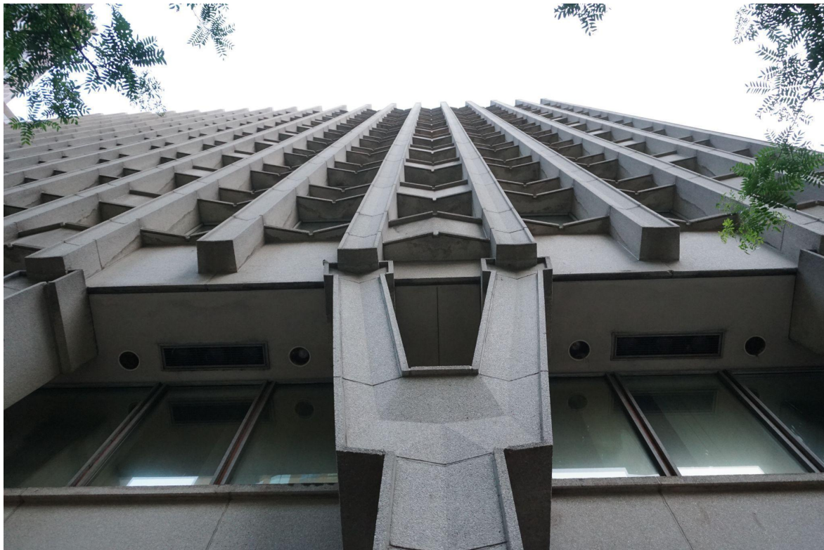
Figure 7. View from below south elevation showing Y-shaped columns, V-cutouts in sills, and concrete columns rising to the cornice, June 2023. Photo credit: Building Conservation Associates.
