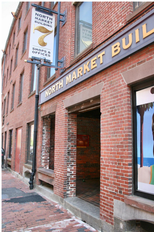
Figure 16. Brick bays converted to integral porch with recessed entry, 7 North Market Building, rear elevation, May 2023. Photo by Kathleen Kelly Broomer.
