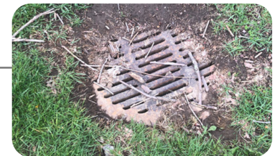
Catch Basins (Varying Condition)
