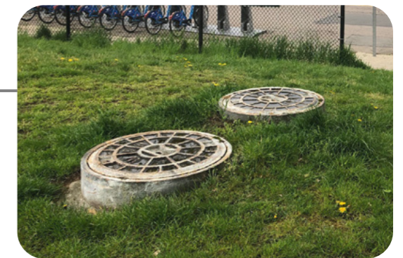
Manhole Covers (Sewer and Drain Lines assumed to be 12+ ft Below Grade)
