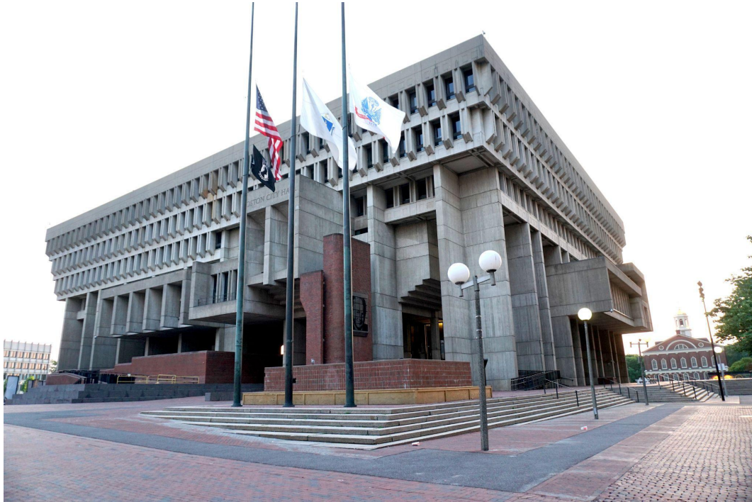
Figure 8. Contextual view of southwest corner with Faneuil Hall in the background at right. (2023)
