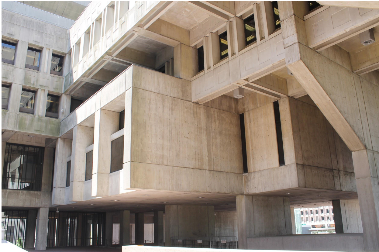
Figure 12. Cantilevered hoods and balconies in the central courtyard. (2018)
