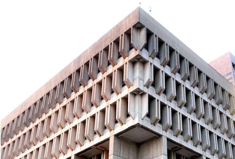
Figure 10. Crown detail (northwest corner) showing alternating windows and fins at upper (administrative departments) levels. (2023)
