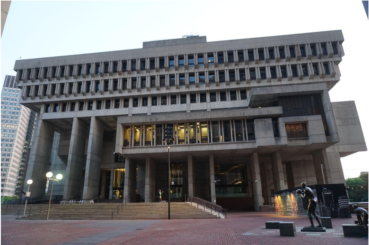
Figure 5. South elevation, June 2023. Photo credit: Building Conservation Associates.
