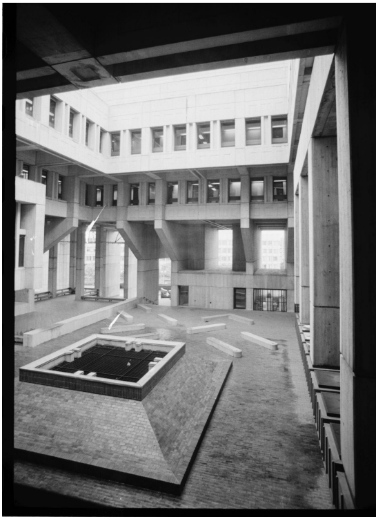
Figure 19. Historical image of central courtyard showing skylight structure at left.
