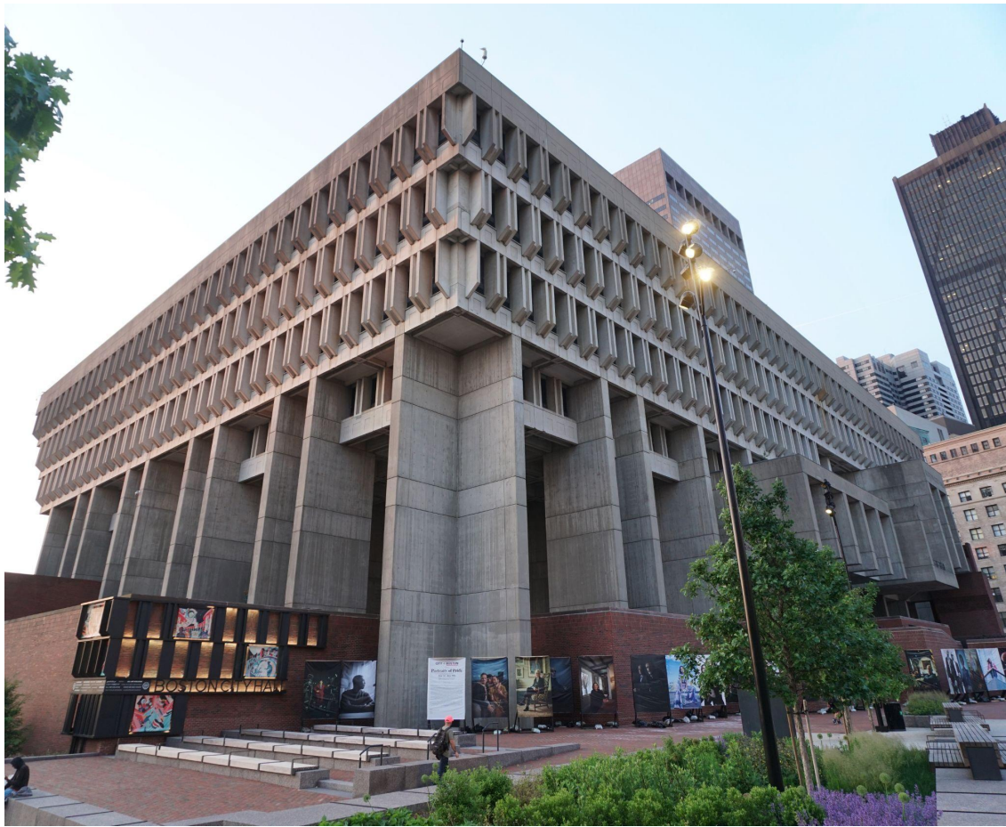
Figure 7. View from northwest, June 2023. Photo credit: Building Conservation Associates.
