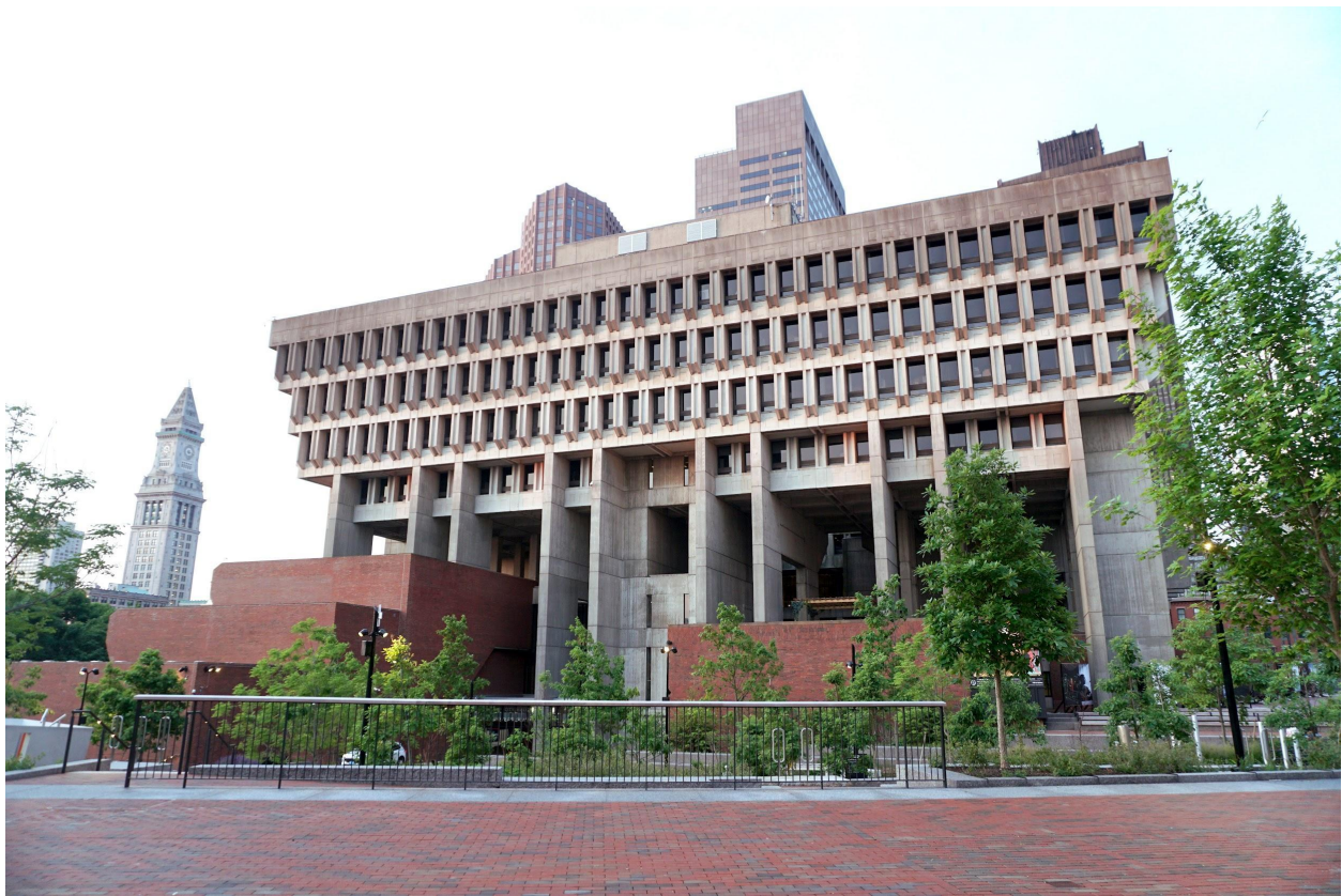
Figure 3. North elevation, June 2023. Photo credit: Building Conservation Associates.
