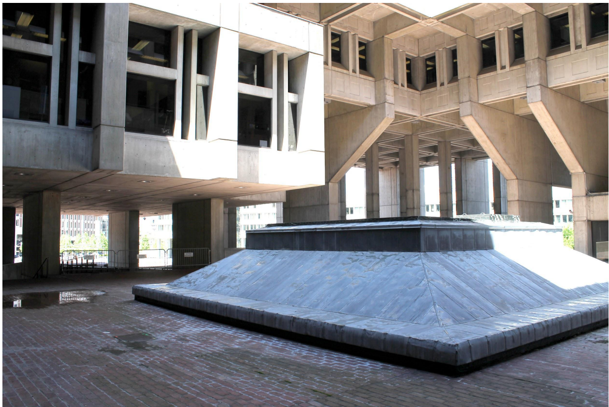
Figure 13. Pyramidal skylight in the central courtyard. (2018)
