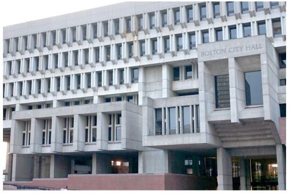
**Figure 11**. Cast-in-place concrete hoods for City Council offices (left) and City Council Chamber (right), June 2023). Photo credit: Building Conservation Associates.
