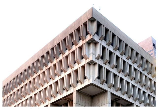
**Figure 10**. Crown detail (northwest corner) showing alternating windows and paired fins at upper (administrative departments) levels, June 2023. Photo credit: Building Conservation Associates.
