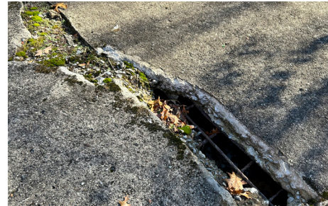
Concrete pavement void, trip hazard
