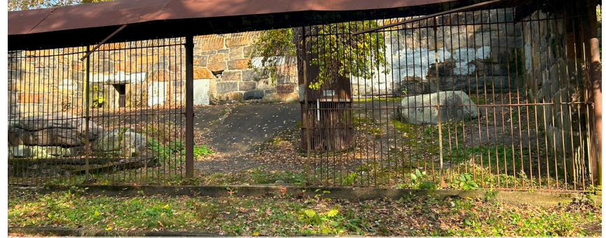
Steep grades, multiple layer of curbing and voids in pavement, trip hazards
