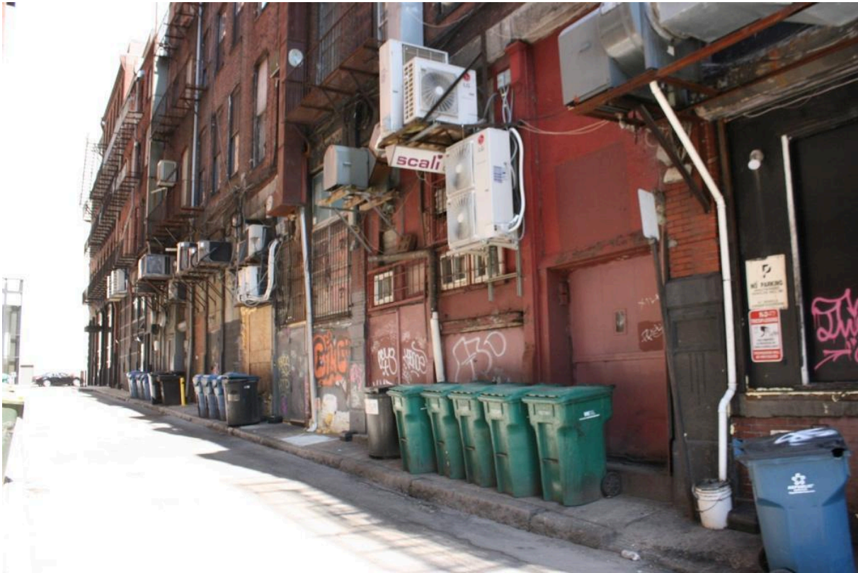
Figure 19. Gridley Street elevations, looking toward High Street. Photograph by Wendy Frontiero, June 2023.
