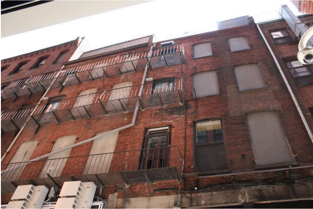
Figure 20. Gridley Street elevations of 123-127 and 129-131 Pearl St. Photograph by Wendy Frontiero, June 2023.
