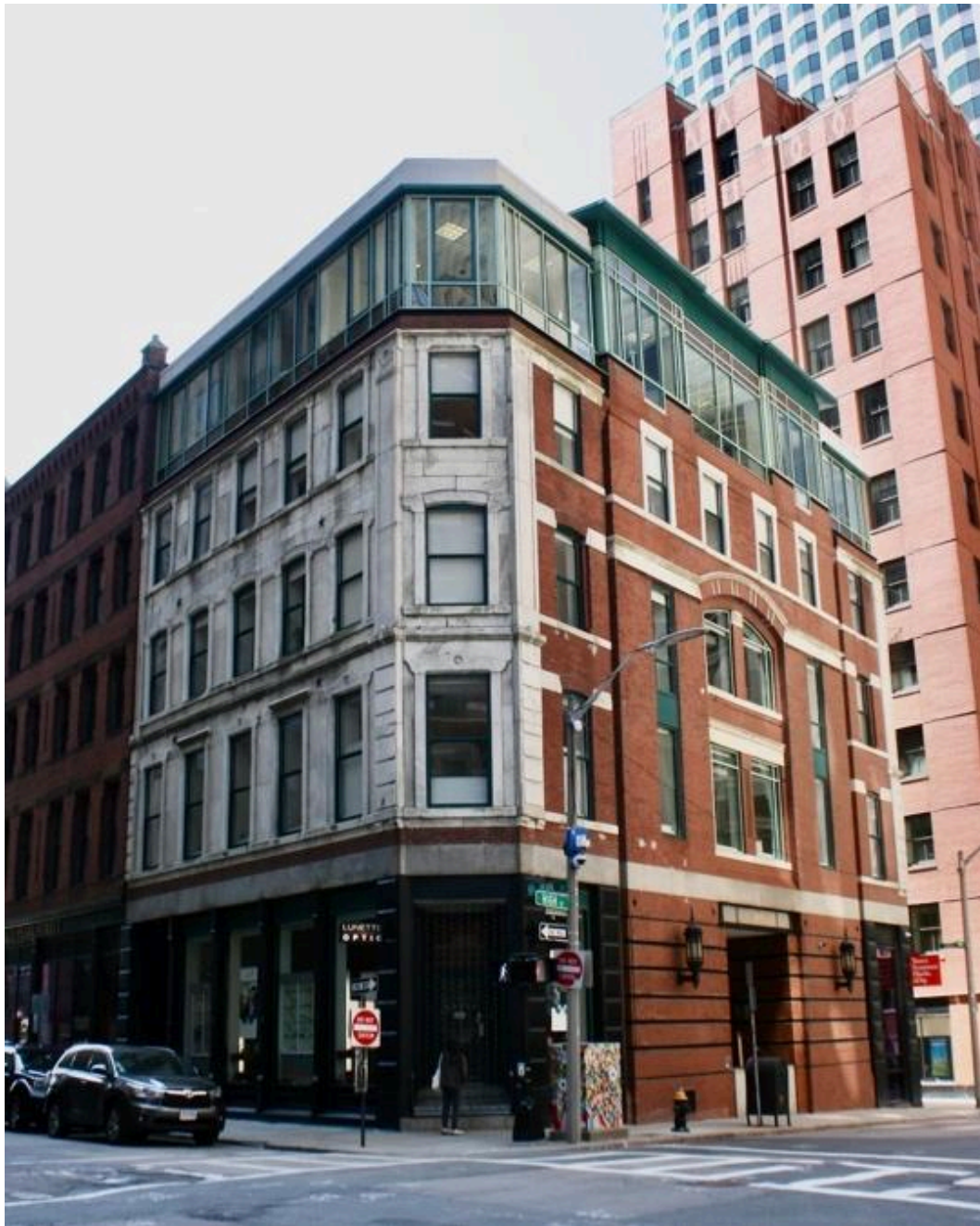
Figure 6. 119 High St.: Pearl Street (left) and High Street (right) façades. Photograph by Wendy Frontiero, June 2023.
