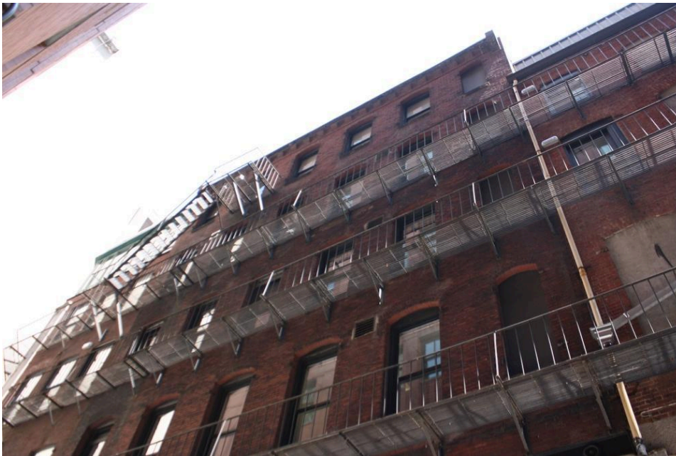
Figure 21. Gridley Street elevation of 115-119 Pearl St. Photograph by Wendy Frontiero, June 2023.
