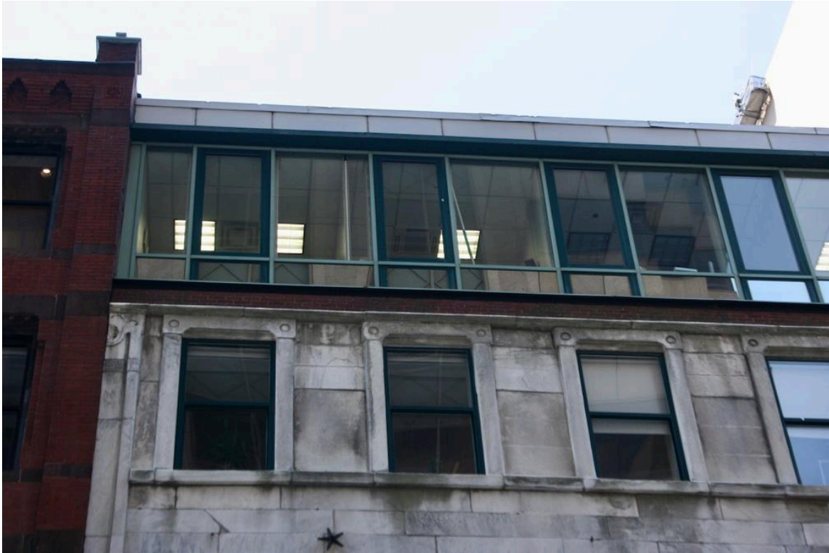
Figure 18. 119 High Street: Penthouse addition. Photograph by Wendy Frontiero, June 2023.
