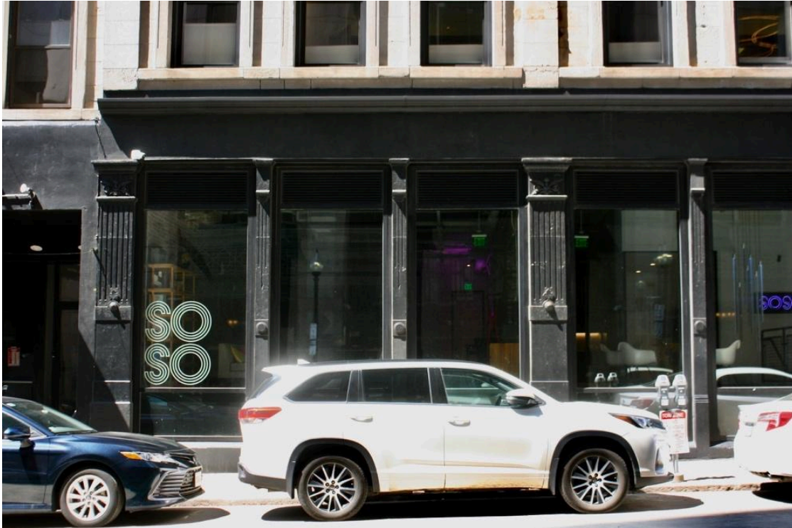
Figure 10. 129-131 Pearl St. storefront. Photograph by Wendy Frontiero, June 2023.
