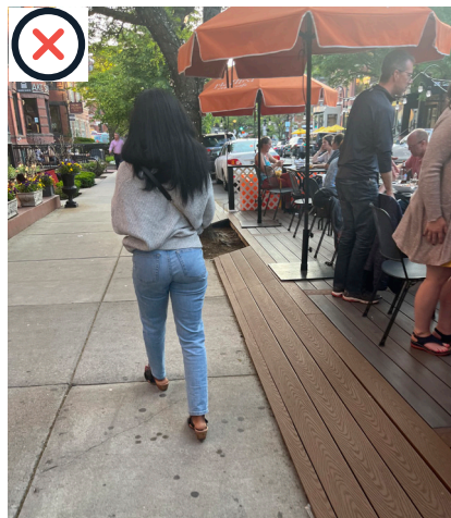
Not allowed! Decked patios must be flush with the sidewalk. No ramps to decked patios.
