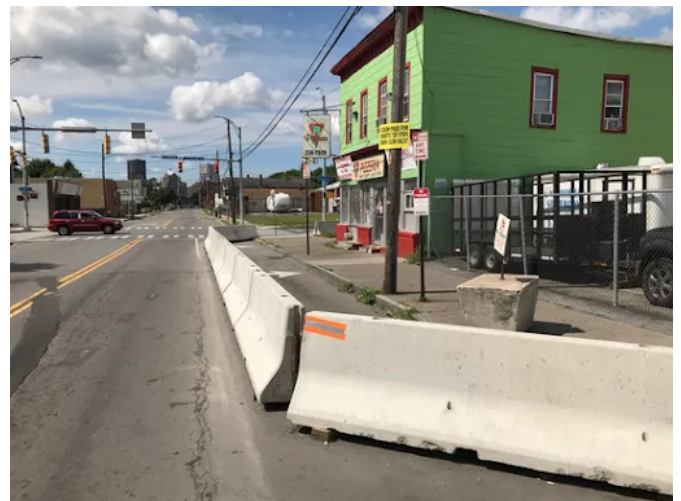
Concrete jersey barrier
