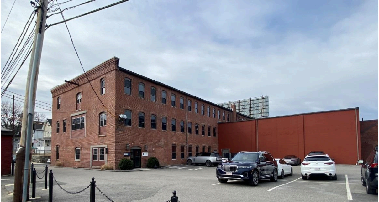
Figure 5. 12 Ericsson St. showing blocked-in window and door openings on the east- and north-facing rear elevations and the concrete-block structure connecting to 12R Ericsson St. Photo by John D. Clemson, March 17, 2023.
