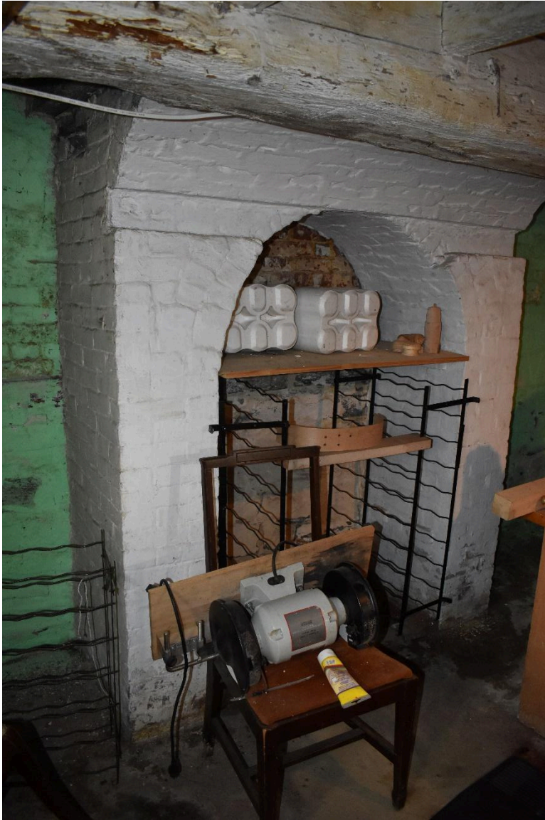
Figure 9. Basement, southwest chimney relieving arch. Photo by The Public Archaeology Laboratory, Inc.
