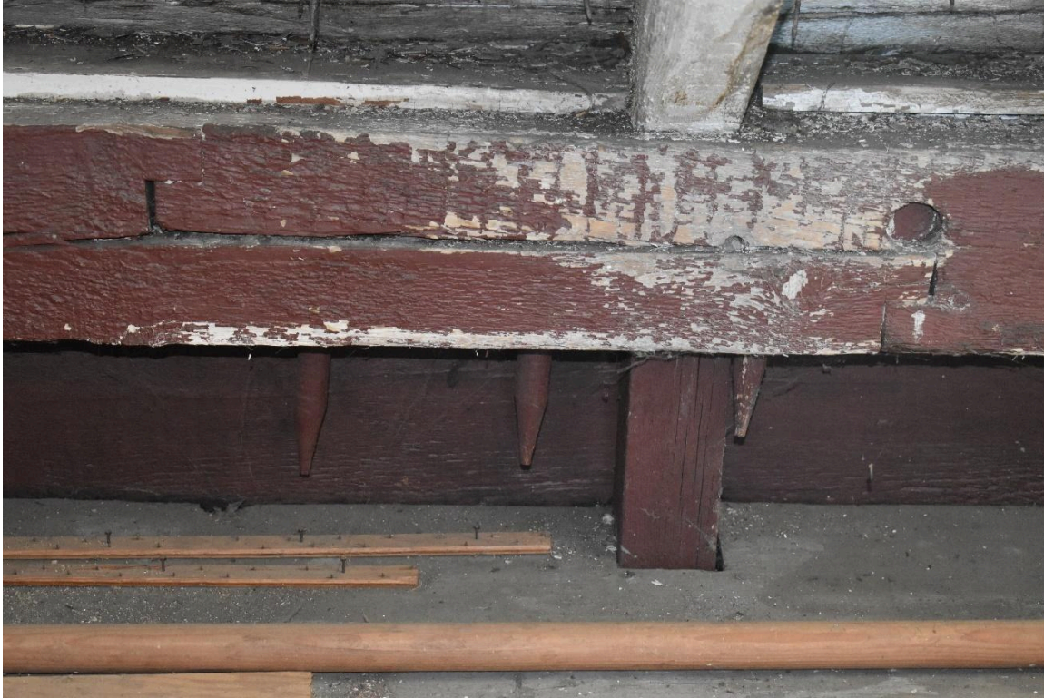
Figure 17. Attic, showing sistered eave plate with dowels, rafter (white), and secondary post (red). Photo by The Public Archaeology Laboratory, Inc.
