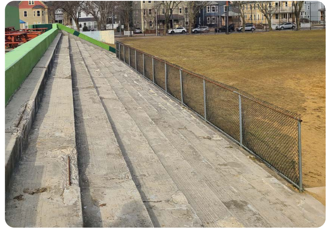
View of Bleachers From Within
