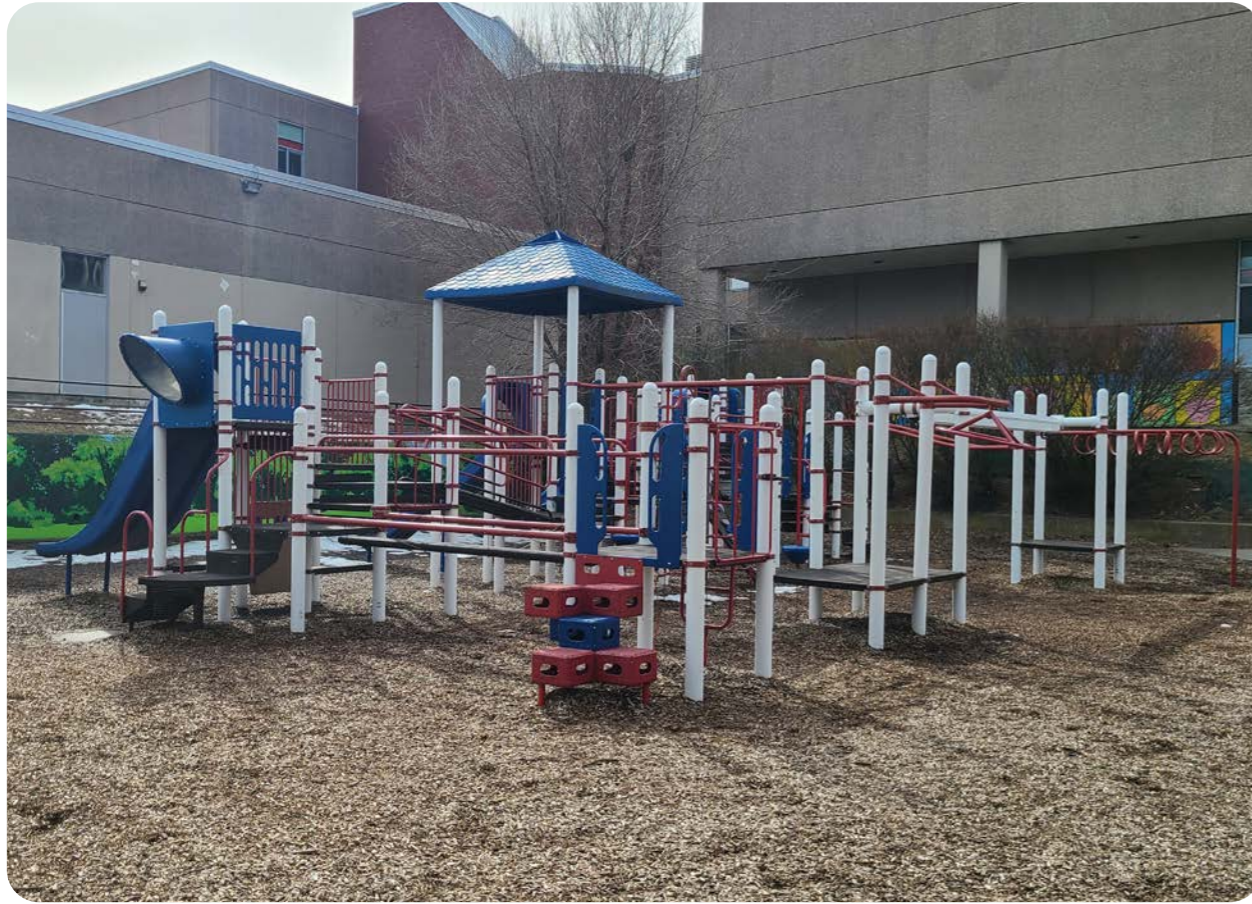
View of Play Structure Looking South West
