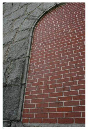
Figure 11. Bricked-up window at the Gate House/Filth Hoist.
