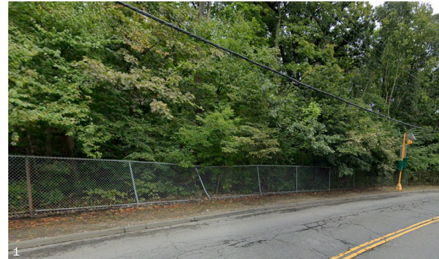
Chain link fence along Williams Street.
