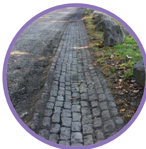
Historic Cobble Gutter
