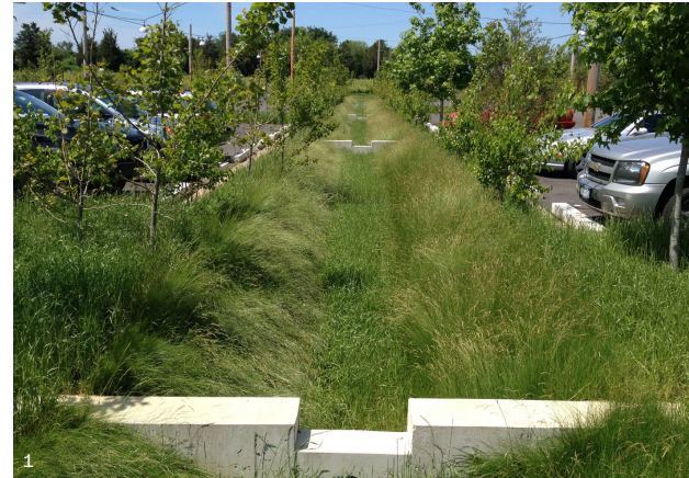
Vegetated swale in the center of parking.
