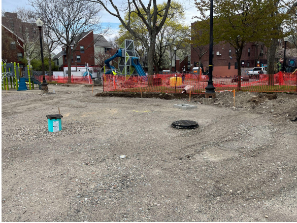
Grading and drainage in the basketball area
