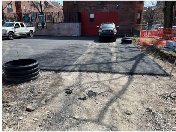
Base course of basketball paving
