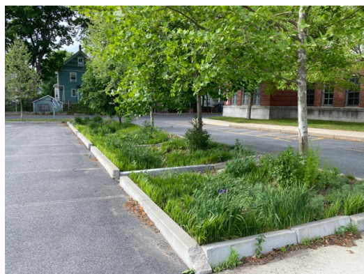
Existing Rain Garden
