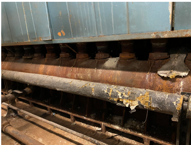
Photos 3 & 4: Existing return headers under the boiler.
