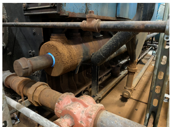
Photos 3 & 4: Existing return headers under the boiler.
