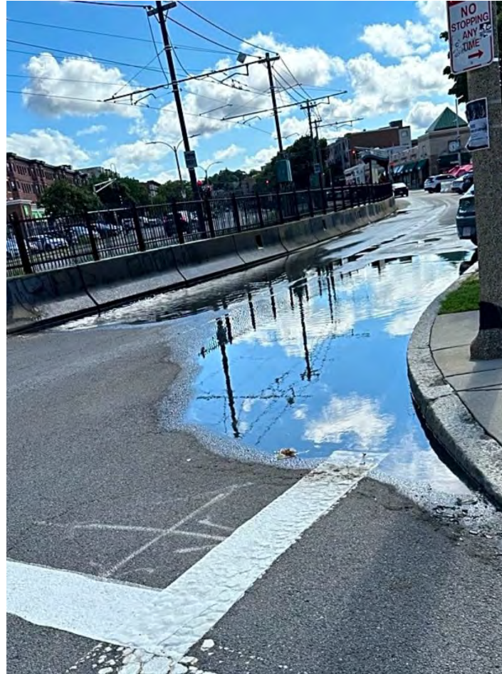
Flooding along Commonwealth Ave in Allston after rain event in January 2025. Road reportedly takes days to drain completely.
