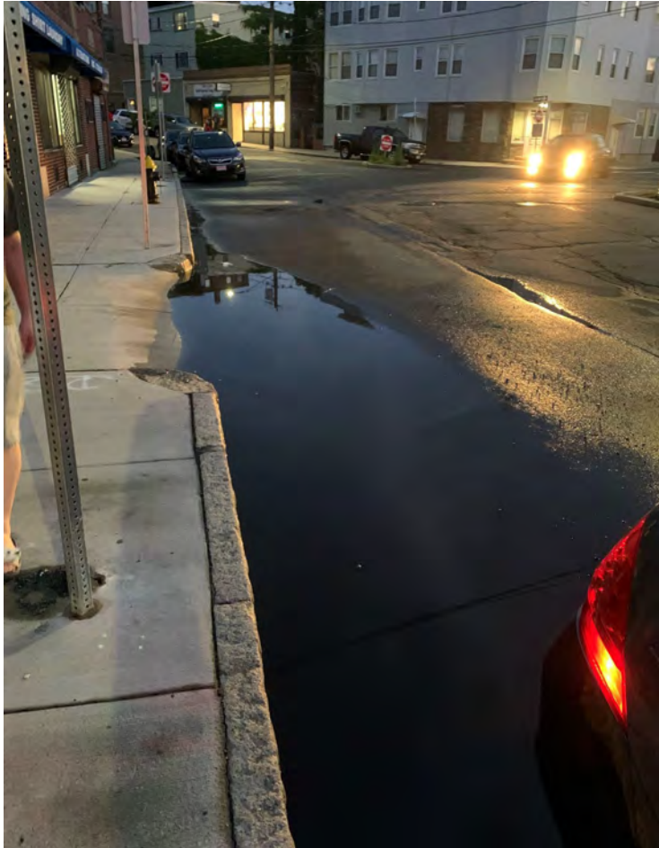
Flooding along Breed St in East Boston in December 2024. Ponding reportedly remains long after rain event.
