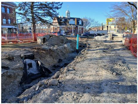
Looking down the future main pathway through the site toward the Washington+Talbot intersection. Here you can see an infiltration trench and new drain work.
