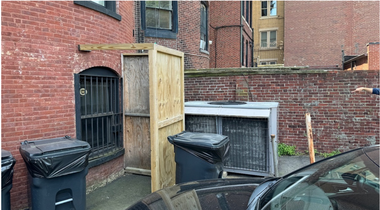
The existing Air-Cooled Condensing Chiller will be removed and replaced.
