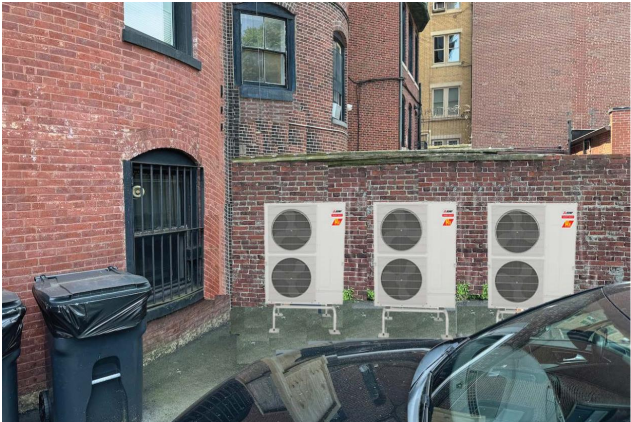
Three new Heat Pumps will provide heating and cooling to the Lower Floor Units of 242 Beacon Street, consuming less energy and generating less noise than the ACCU being replaced.
