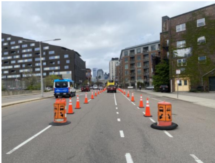
Figure 1: Northbound Dorchester Ave Coned Bus Lane between W Fourth St and A St during May Red Line Diversion
