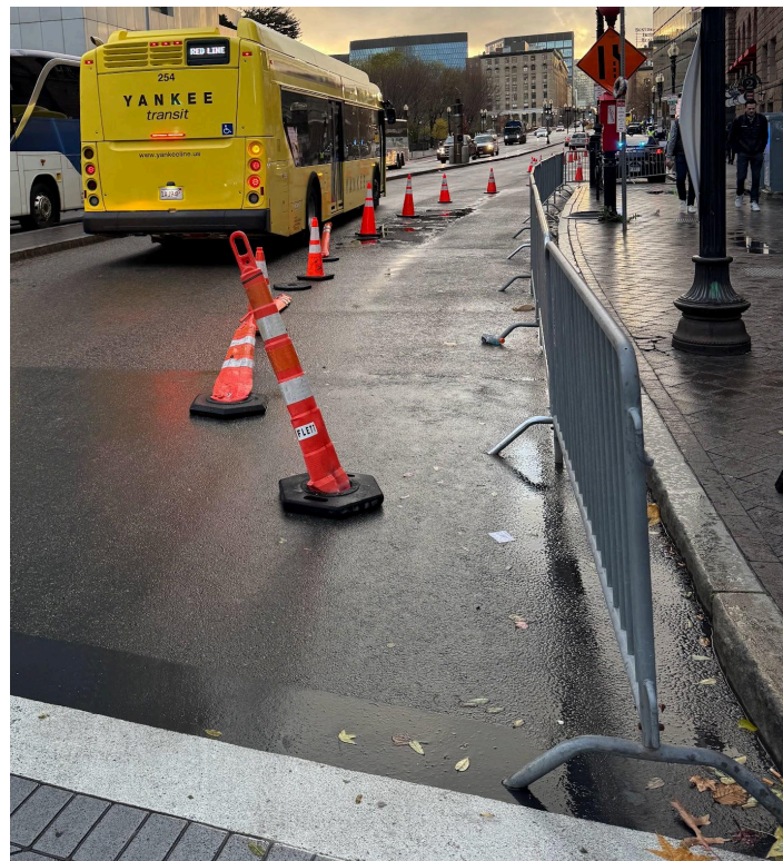
Figure 11: BPD metal barriers provided for November Red Line Diversion to discourage rideshare PU/DO
