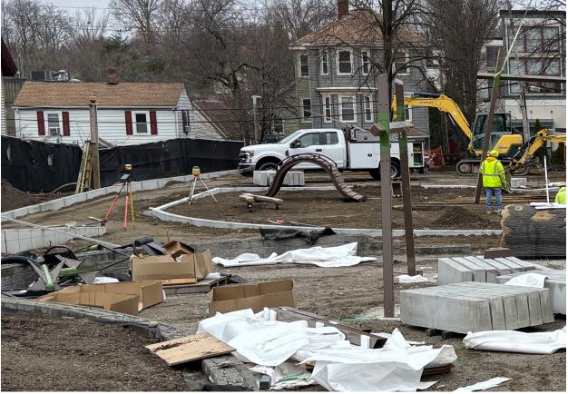
The precast concrete curbs and part of the swings have been installed!
