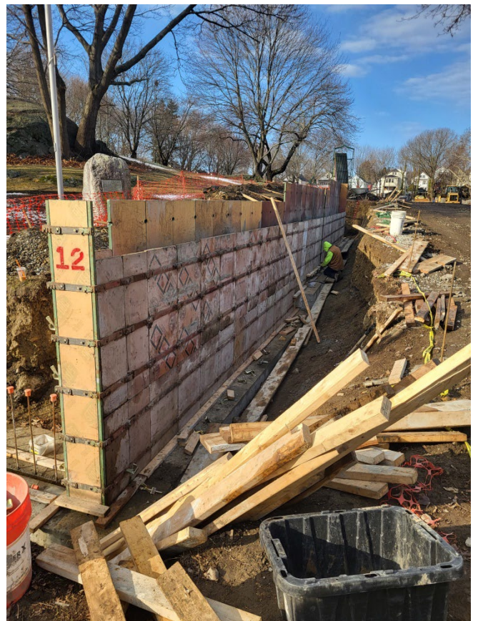
Formwork in place to pour the concrete wall near the entrance at Washington Street. Only about 18" of the wall will be visible in the final condition
