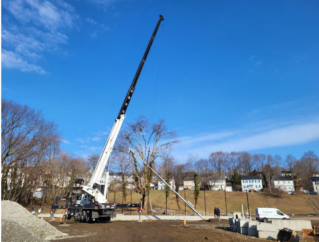
A crane lifting the light pole in place for the basketball court lighting
