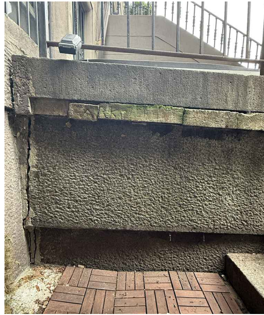
VIEW OF GRANITE AT EXISTING WALL (CONDITION FOR REUSE TBD)
