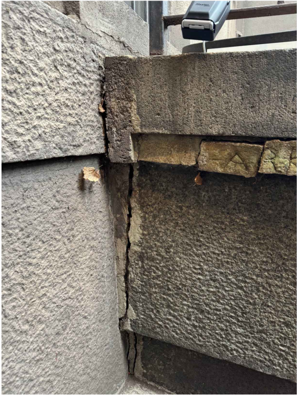
VIEW FROM LANDING (GARDEN LEVEL ENTRY) DETERIORATION & RETAINING WALL FAILURE - DISLOCATION OF EXISTING STRUCTURAL WALL FROM PERPENDICULAR FOUNDATION IS CONTRIBUTING TO WATER/MOISTURE INFILTRATION AT LOWER LEVEL UNIT. OVERGROWN TREE ROOT SYSTEM & UNEVEN/ UNSUSTAINABLE GARDEN GRADE ALSO A LIKELY CONTRIBUTOR, PER STRUCTURAL ENGINEER'S ASSESSMENT.
