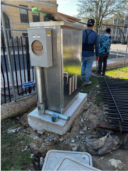
Electrical cabinet installed
