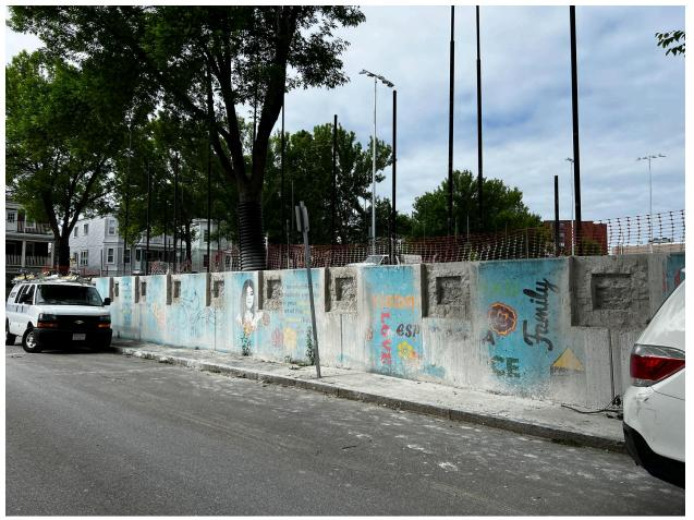
Holes have been cut in the perimeter site walls to make room for the soil nails which will secure and stabilize the walls.
