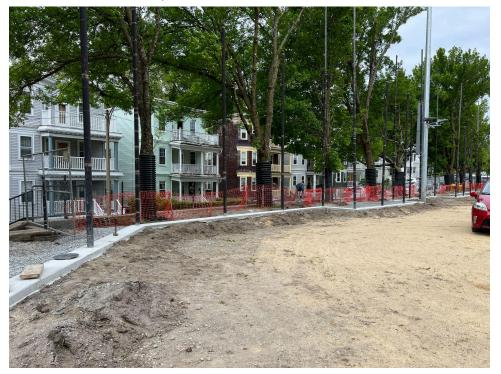
$Concrete\ mow\ strip\ below\ the\ chain\ link\ fence\ has\ been\ installed.$
