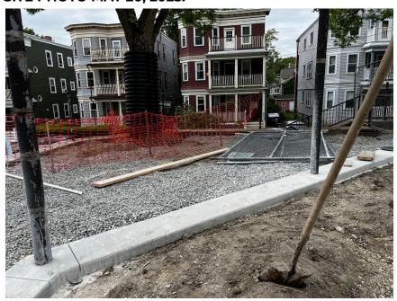
The gravel base for the porous paving has been installed.
