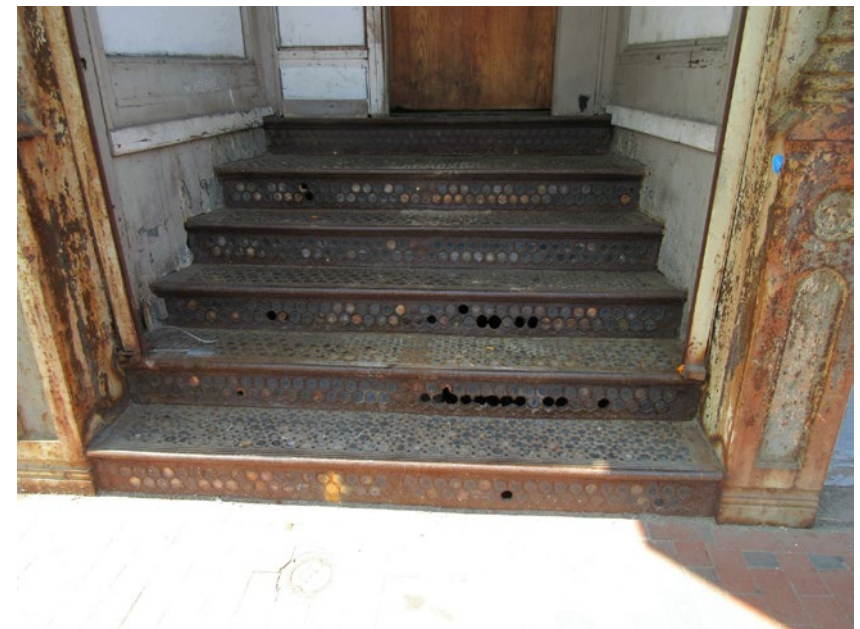
CAST IRON STAIRS WITH PRISM LIGHTS
