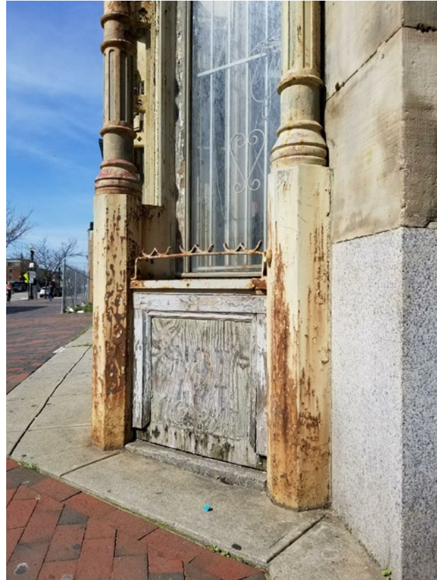
BOTTOM OF CAST IRON STOREFRONT
