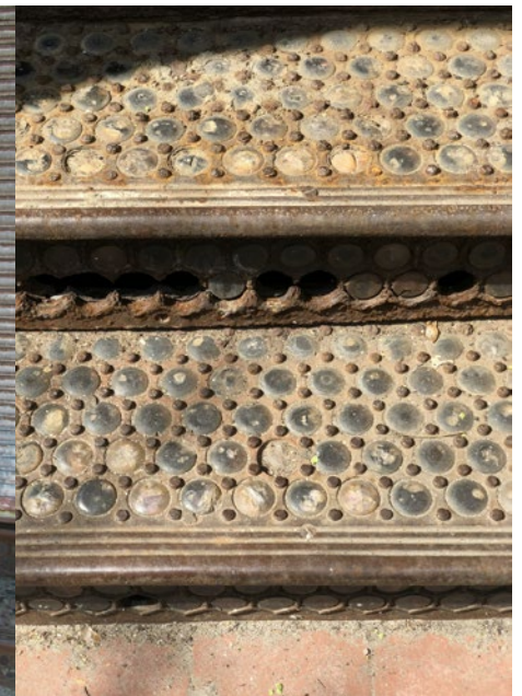
CLOSE-UP OF CAST IRON STAIR
