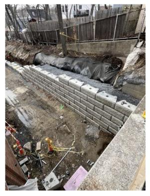
New site retaining wall at North side and underground site work adjacent to Sycamore St.
