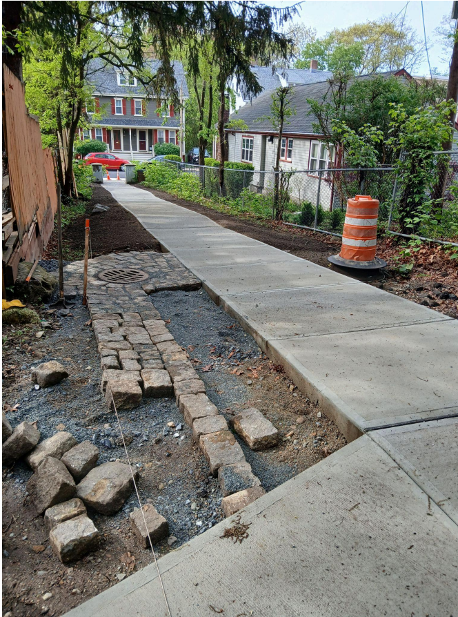
The renovated entrance at Richmond Street and the layout of the new granite cobblestone swale that leads to the stormwater catchbasin.
