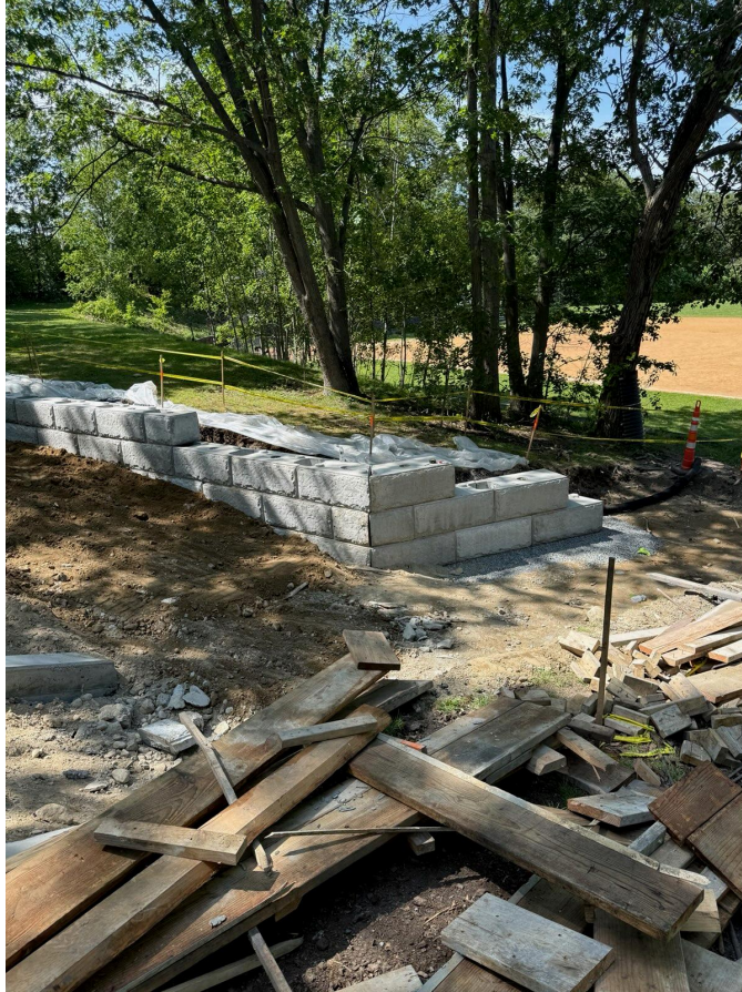
Progress on the segmental block retaining wall near the softball field.
