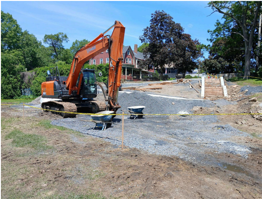
Work began on the new concrete ramp and stairs at the Richview Street entrance.
