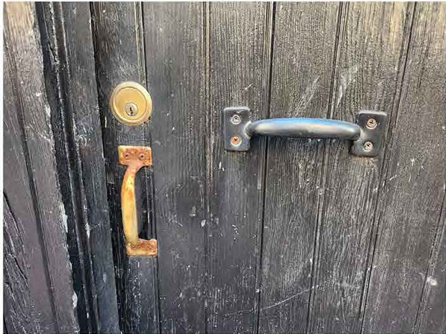
Existing Gate Hardware
