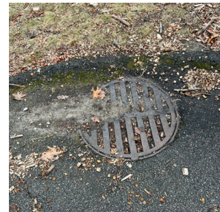
EXISTING CLOGGED DRAIN
