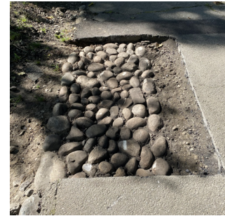
EXPOSED COBBLESTONE SWALE
