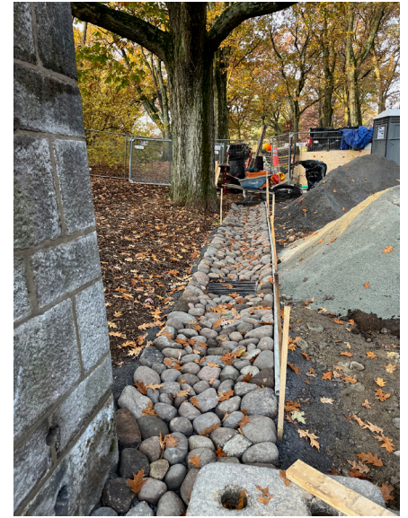
RESTORED COBBLESTONE SWALE W/ DRAIN COVER
