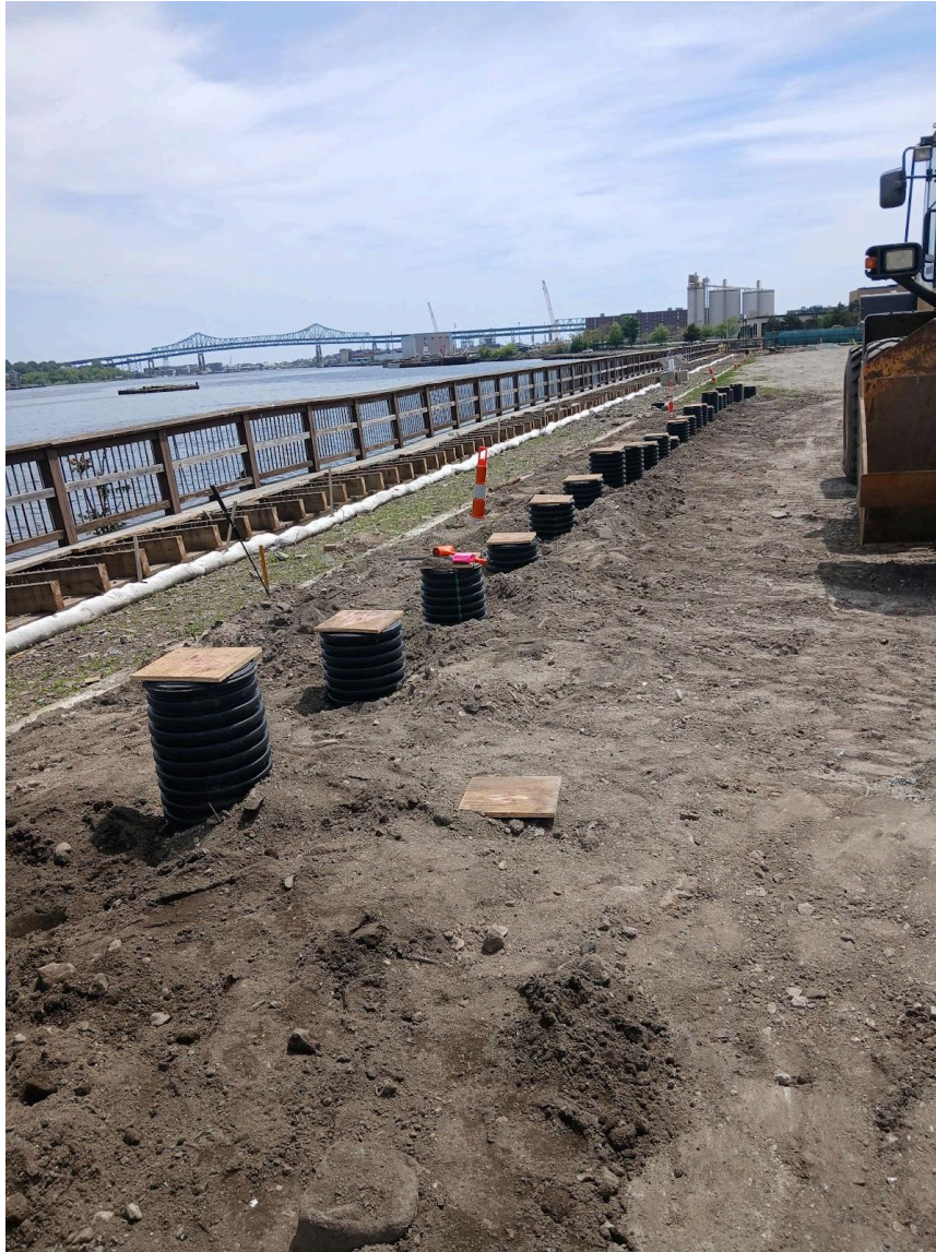
Pre-dug sleeves at future micropile locations along the gas main line.
