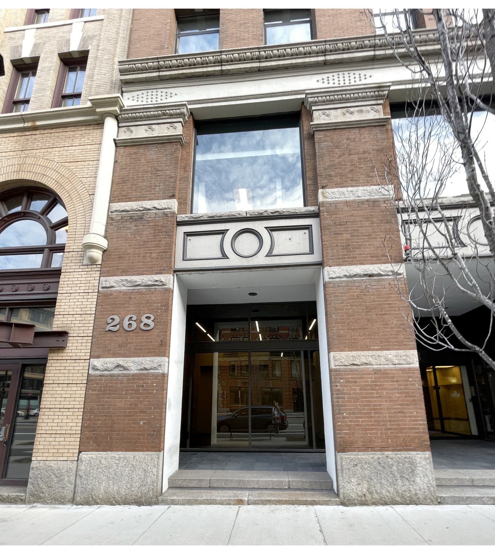
EXISTING ARCADE ARCHWAY ADJACENT TO ENTRY W/ ADDRESS SIGNAGE
