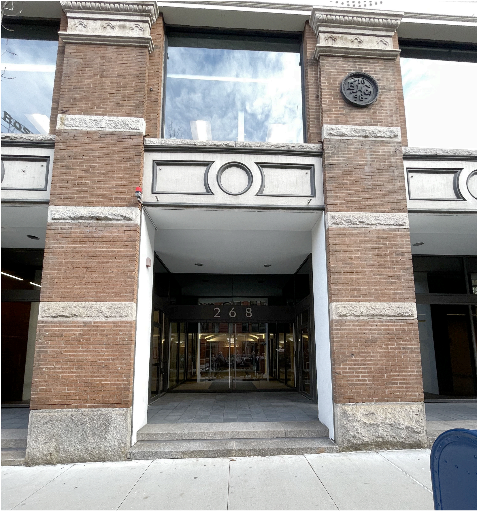
EXISTING ENTRY ARCHWAY
