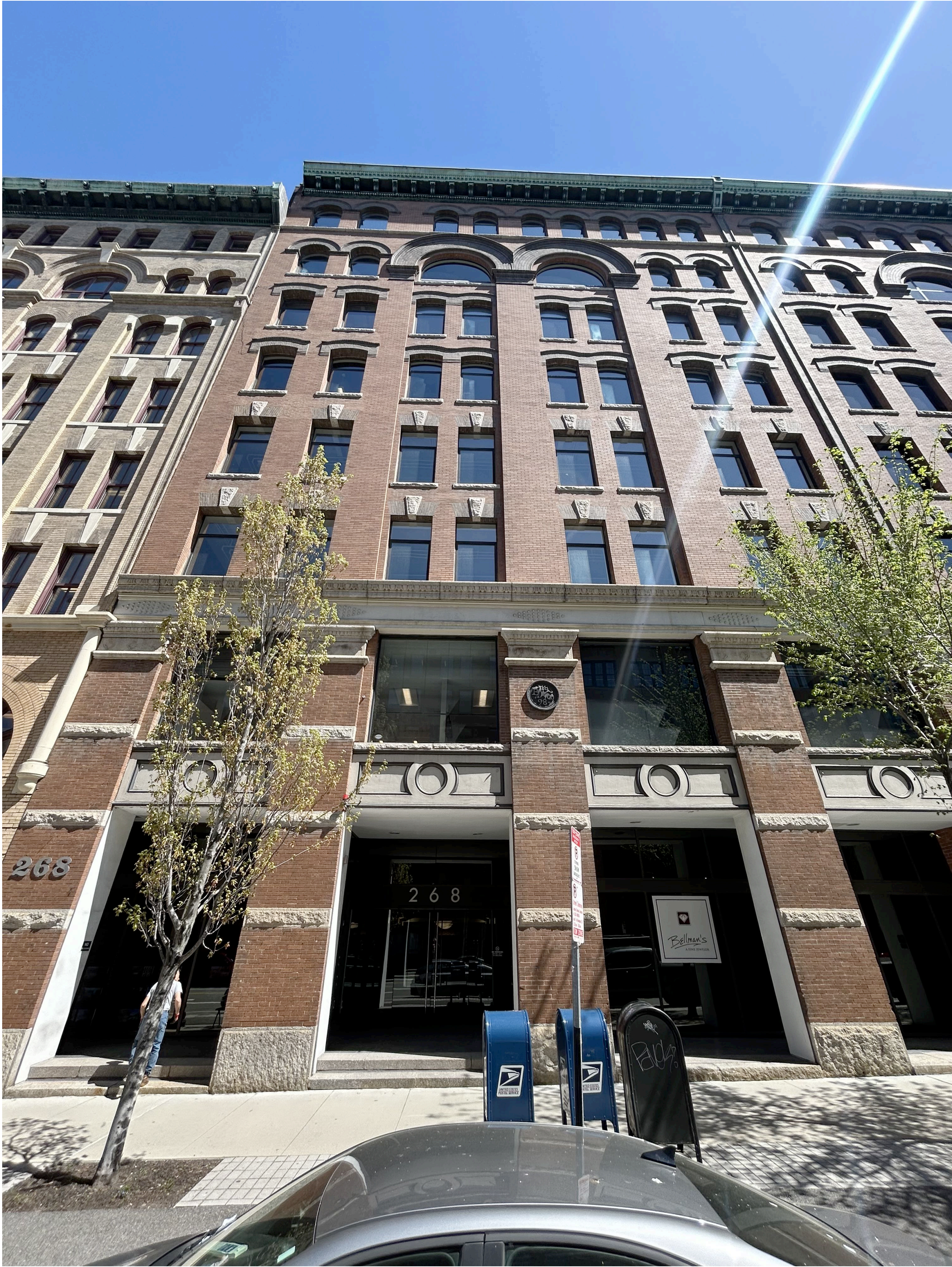
EXISTING EXTERIOR FACADE
