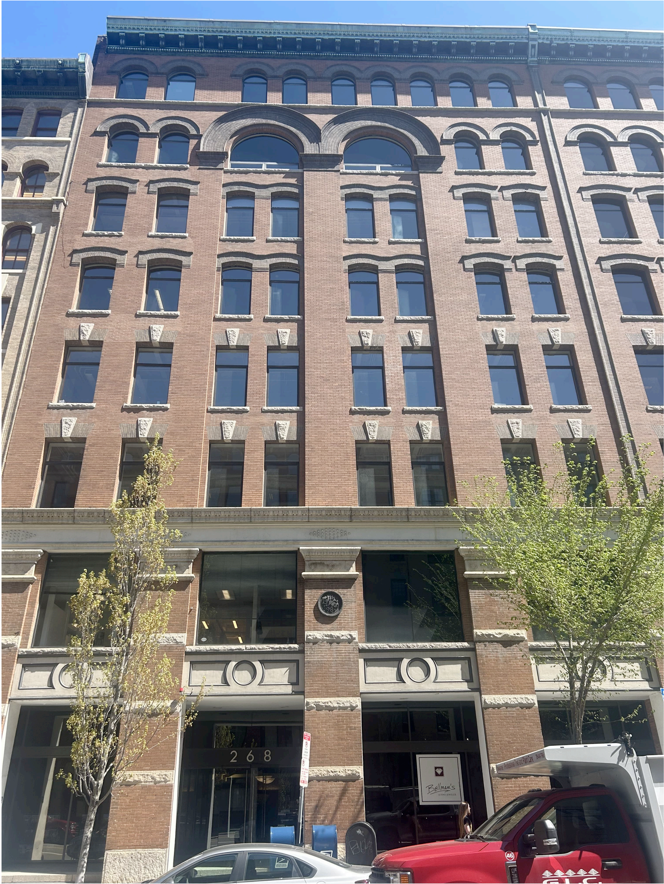
EXISTING EXTERIOR FACADE
