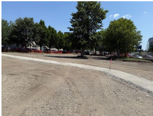
Rough grading and layout
